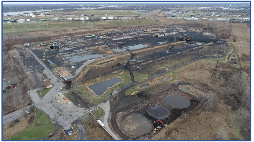
Fall 2022 after view from southwest corner
